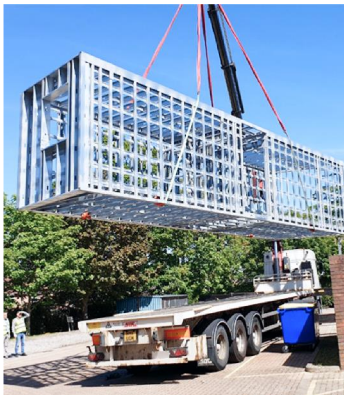
METAL FRAME PRODUCTION
